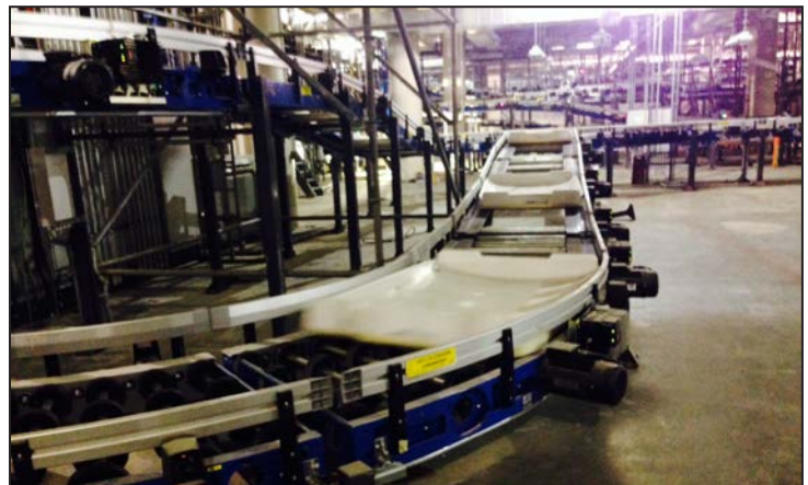
Above: Tote-Tray conveyor system
