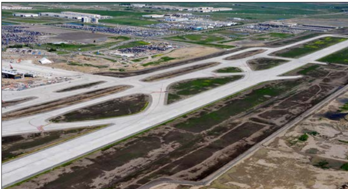
Above: Runway Development Project complete
