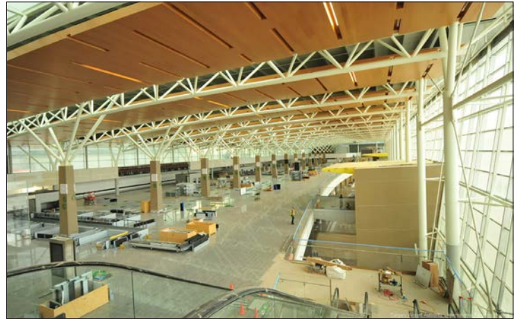
Above: Departures Check-in Hall of the IFP
