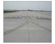
A Maximum Wingspan Marking is information denoting the maximum aircraft wingspan allowed in that area. The wingspan of an aircraft is always measured in a straight line, from wingtip to wingtip, independently of wing shape or sweep. The Maximum Wingspan Marking is located across the surface of a Taxiway/Apron Taxiway centerline.
