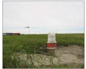
Runway Edge Lights are single white lights used along the edges of Runways. Runway 17L-35R has lights with a two-color head. The last 600 meters (2000 feet) of lights are yellow on one side and white on the other. The yellow lights act as a warning to pilots that the Runway is about to end.
