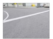
STOP Lines are a single solid white line and are used to indicate a MANDATORY STOP to the driver. A STOP sign is typically installed at a STOP line. All drivers are expected to STOP at a STOP line whether or not there is a STOP sign.
