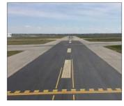
The center of a Runway is marked with broken white lines composed of several lines close together. Each group is 30 meters in length with 30 meters in between.
