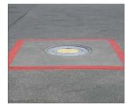
A red square indicates an underground fuel valve that is used when refueling aircraft. Parking is not allowed over or within 2 meters of Fuel Isolation Valve Chambers (Fuel Vaults).
