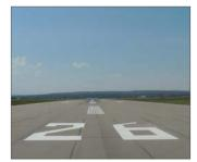
Each end of a Runway is numbered with the Runway Heading, in tens of degrees, corresponding to the direction of the Runway in relation to a magnetic compass. The compass of an aircraft will read 260 degrees when approaching the end of a Runway marked with the number 26. The numbers are painted in white and face towards the end of the Runway. YYC Runway headings are 08, 11, 17R, 17L, 26, 29, 35R, and 35L.
