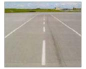
Vehicle Service Roads (VSRs) are indicated by two solid white lines at least 7.5 meters apart with a single broken center line. VSRs may be two-way traffic, or one-way traffic. (<u>Ref. 6.7</u> for VSR right-of-way rules)
