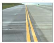
Taxiway Edge Lines consist of double solid yellow lines. The double solid yellow lines along with a series of single blue lights on a Taxiway are used to indicate the edge of the usable portion of the Taxiway. Paved surfaces outside the lines are not designed for aircraft.
