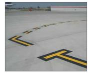
Aircraft Lead Out Lines are a single broken yellow line and are used to guide the aircraft as it taxis out of its Ground Loading parking position. This is the route an aircraft takes when leaving a Ground Loading Operational Stand under power.
