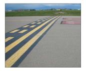
Runway Holding Position markings consist of two solid and two broken yellow lines across the width of a Taxiway with the broken lines closest to the Runway to indicate a Runway holding position.
