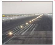
Runway Center Line Lights are inset white lights that run along the Runway center line with directional red lights at the extremities of the Runway. The last 300 meters of the center line lights are red, and the lights between 300 meters and 900 meters alternate between red and white. This system of red and white lights act as a warning to pilots that the Runway is about to end. Runway Center Line lights are located only on Runway 17L-35R.
