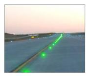
Taxiway Center Line lights are green lights co-located with the Taxiway Center Line. Taxiway Center Line lights are located on the East airfield and on the Apron Taxiway on Apron I near the ITB. Taxiway Center Line lights indicate the location of the Taxiway center line as well as permission for aircraft to progress along the Taxiway. These lights are used during reduced and low visibility operations for aircraft movements. (Ref. 8.9)
