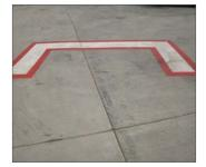
A Bridge Staging Box is a white or red U-shaped marking and is used to indicate where the bridge wheels may be pre-positioned, while still providing clearance for specific aircraft entering the operational stand. The outer red line indicates No Parking in this area.
