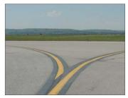
A single solid yellow line located on an Apron. The Apron Taxiway is a portion of an Apron designated as a taxiway providing a through taxi route across the Apron. The Aircraft Stand Taxilane is a portion of an Apron providing access to aircraft stands. The nose wheel of the aircraft is centered on this line to ensure that the main wheels are on the pavement and the wings do not make contact with any known obstructions.
