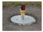
In addition to single blue lights on the edge of most Taxiways, one-way Taxiways have half-blue and half-red lights. The red half of the lights are seen when traveling on the Taxiway in what would be the wrong direction for aircraft.
