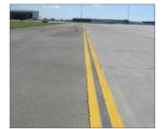
Apron Edge Lines are double solid yellow lines. Apron Edge Lines and the co-located single blue lights. Apron Edge Lines and the co-located single blue lights are used to indicate the edge of an Apron and the edge of a Taxiway. Paved surfaces outside of the Apron Edge Lines are not designed as weight bearing surfaces adequate for aircraft. Vehicles and equipment parked or operating outside of the Apron Edge Lines are NOT guaranteed safe clearance from aircraft.
