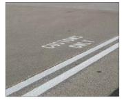
Lease Lines are two white (or yellow) parallel lines with the word "Lease" (or a company name). Lease Lines are used to outline the area of an Apron surface that has been leased to a company. An AVOP is not required for company employees or company authorized persons to operate vehicles, equipment or aircraft inside the leased area.
