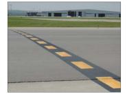
A Taxiway Intersection Marking consists of a single broken yellow line (e.g. at the intersections of Taxiways C and J). A Taxiway Intersection Marking is located at such a position that a holding aircraft or vehicle would not protrude into the intersecting taxiway strip. An aircraft or vehicle instructed to hold short of a Taxiway Intersection Marking must remain behind this line. These markings are co-located with Location/ Directional signs.
