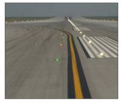
Rapid Exit Center Line lights are a series of inset alternating green and yellow lights. Rapid Exit Center Line lights mark the high-speed exits from a Runway to a Taxiway. The inset lights are two-directional so that the alternating colours show only when exiting the Runway and only if the lights are green from the Taxiway onto the Runway. Rapid Exit Center Line lights are located only on Runway 17L-35R.
