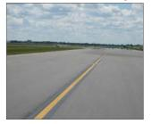
The Taxiway Center Line is a single solid yellow line on a Taxiway and is used to provide guidance for aircraft to taxi from the Runway center line to a point on the Apron where aircraft operational stand markings begin. The nose wheel of the aircraft is centered on this line to ensure that the main wheels are on the pavement and the wings will not make contact with any known obstructions.
