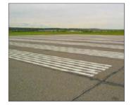
Threshold Markings indicate the beginning of the usable part of the Runway for aircraft landing. Threshold Markings are a series of solid white lines in groups that run parallel to the length of the Runway. The number of lines in a group and the total number of groups of lines is dependent on the width of the Runway.
